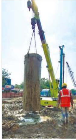
Casing Removal
